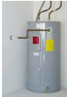
What happens? When an electric or gas water heater isn't maintained or just gets old, it can develop a sediment (rust, minerals, etc.) buildup in the bottom of the tank. When this happens, it can cause the hot water to turn a brownish color and even cause odor issues.
